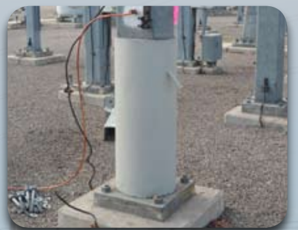
Remove ratchet straps & paint jacket (if desired)
