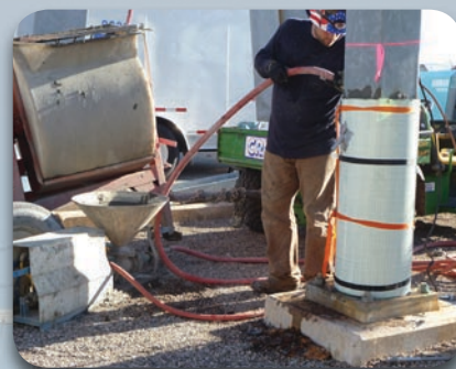
Fill the annular space with grout & vibrate
