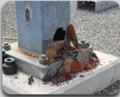
Corrosion-damaged column
