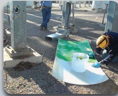
Cut a piece of PileMedic™, apply epoxy & wrap ...
