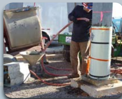
Fill the annular space with grout & vibrate
