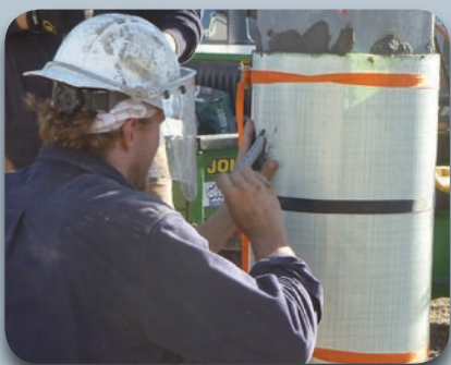
Hold shell together w/ ratchet straps & insert drain pipe
