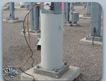
Remove ratchet straps & paint jacket (if desired)
