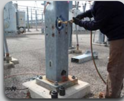
Cut an opening at 30-inch above grade
