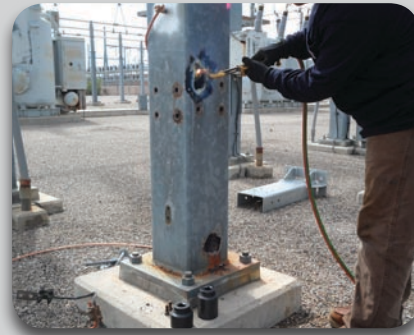
Cut an opening at 30-inch above grade
