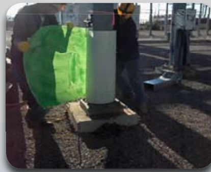
... around the column to create a 36-inch high shell
