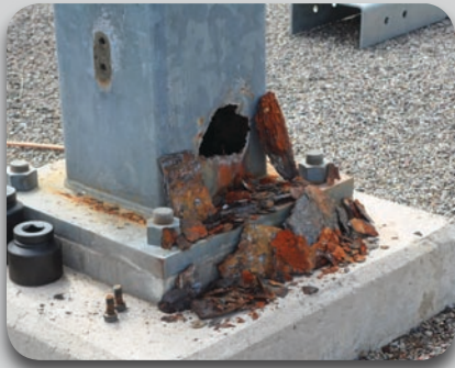
Corrosion-damaged column
