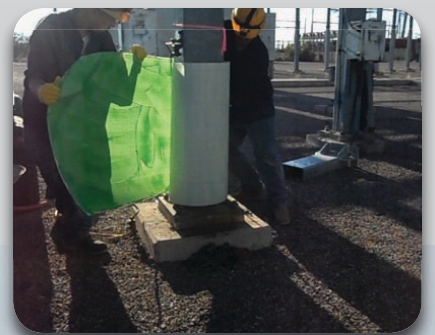
... around the column to create a 36-inch high shell
