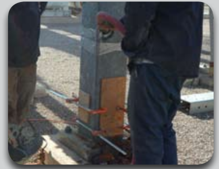
Fill the inside of the column with grout
