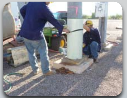
Use ratchet straps to support shell temporarily
