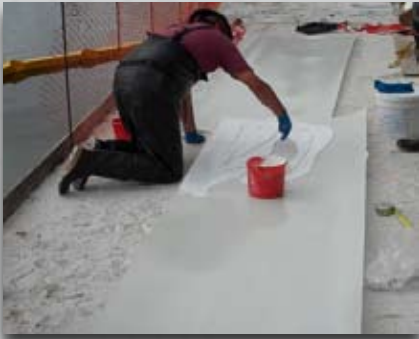
Mix QuakeBond™ 220UR (Underwater Resin) and apply QuakeBond™ 220UR to the back of PileMedic™ with a thickness of about 30-40 mil
