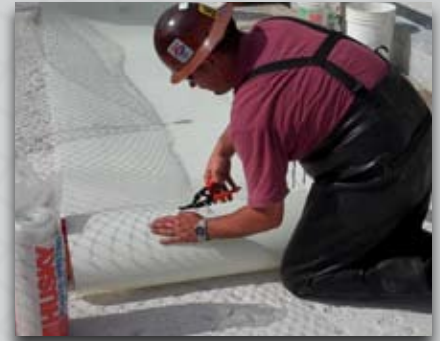
Cut PileMedic™ sheet to desired size
