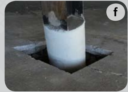
a. Corrosion-damage b. Apply epoxy to PileMedic™ c. Wrap PileMedic™ around column or pile to create a cylindrical shell d. Temporarily support shell w/ ratchet straps e. Fill annular space with grout f. Remove ratchet straps & paint jacket (if desired)
