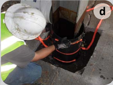
a. Corrosion-damage b. Apply epoxy to PileMedic™ c. Wrap PileMedic™ around column or pile to create a cylindrical shell d. Temporarily support shell w/ ratchet straps e. Fill annular space with grout f. Remove ratchet straps & paint jacket (if desired)
