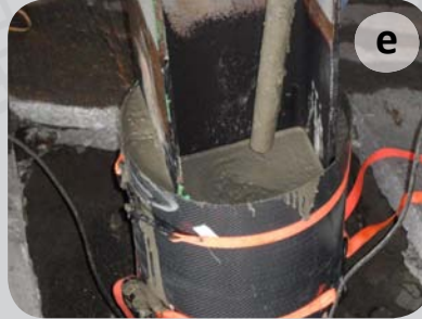
a. Corrosion-damage b. Apply epoxy to PileMedic™ c. Wrap PileMedic™ around column or pile to create a cylindrical shell d. Temporarily support shell w/ ratchet straps e. Fill annular space with grout f. Remove ratchet straps & paint jacket (if desired)
