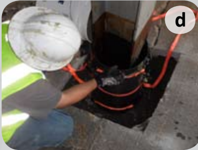
a. Corrosion-damage b. Apply epoxy to PileMedic™ c. Wrap PileMedic™ around column or pile to create a cylindrical shell d. Temporarily support shell w/ ratchet straps e. Fill annular space with grout f. Remove ratchet straps & paint jacket (if desired)
