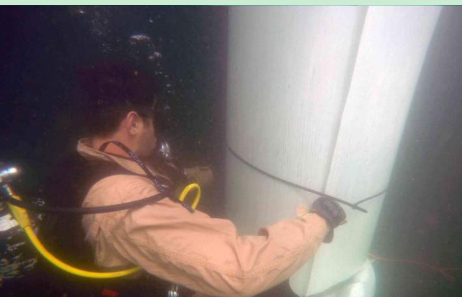
Diver Secures Laminate with Zip Ties
