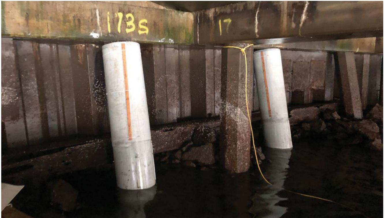
**T**he current repair work — scheduled for completion at the end of 2017 — involves the retrofit of 40 prestressed driven piles of varying length located under T-18. No shutdown of service was needed during repair, with more than half of the piles 30 feet or longer, and in varying degrees of water submersion.
